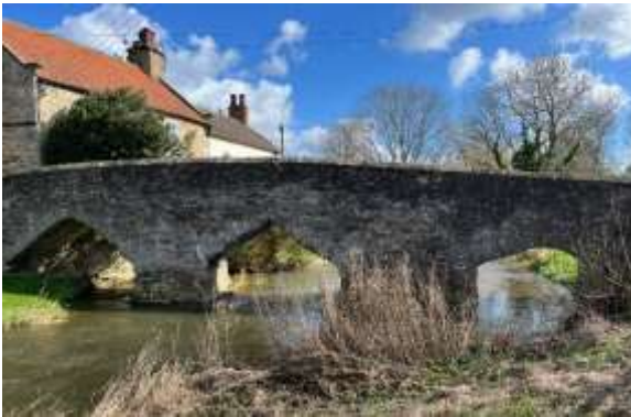
Packhorse bridge at Aldborough St John
